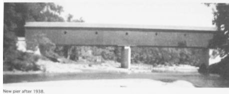
New pier after 1938.
